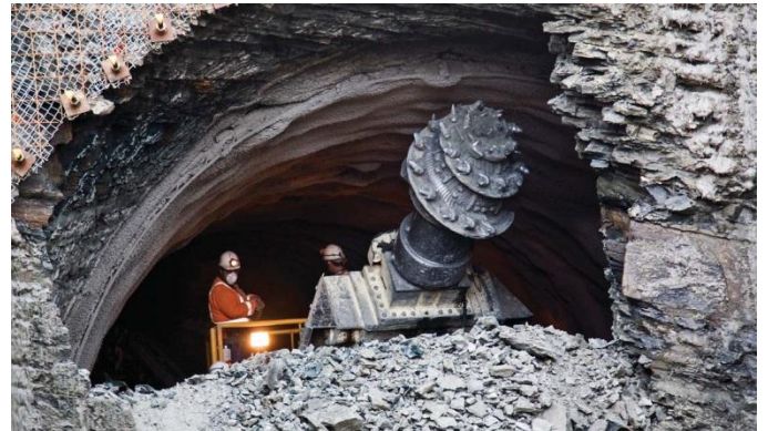
Breaking through to the otherside of Johnstone's Hill
